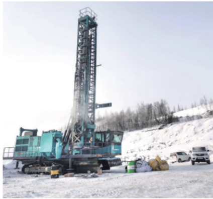
Yakutsk, Russia-SWDR250 roller-bit hole drilling rig
